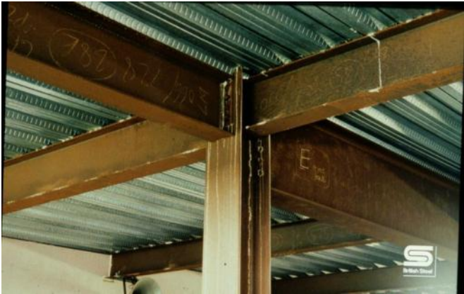
Beam-to-column connection
