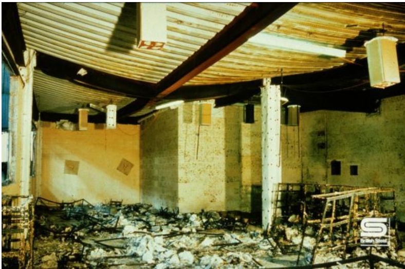
Secondary beam deflection 640 mm
