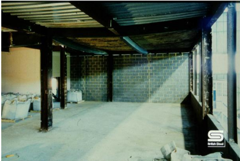
Deformation of the floor slab
