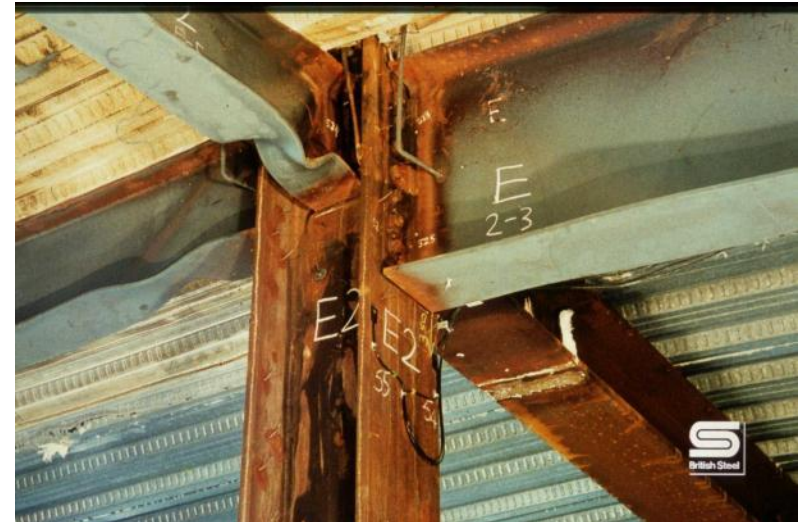
Beams around the fire protected column
