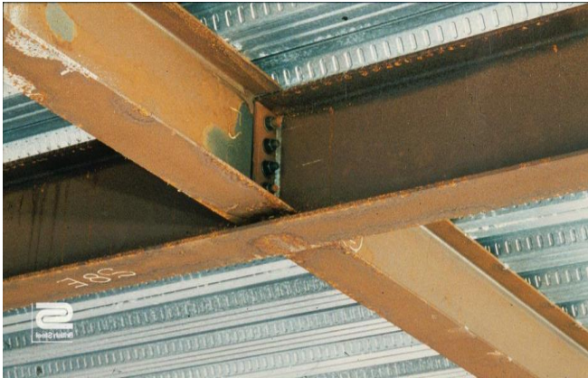
Beam-to-beam connection
