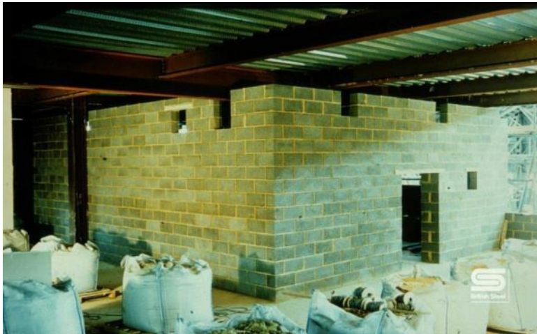
Walls of the fire compartment
